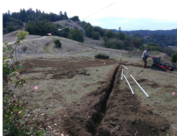
buried 33' wire radials for 40 meter 1/4\lambda . Feedline trench in foreground.
