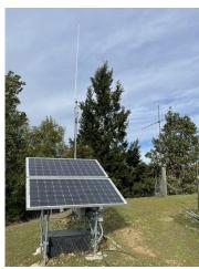
To increase the available power and more rapidly recover from deep discharges, I replaced the 50w panels with two, 175w @ 44 volt panels, wired in series, and installed a 100 volt/30 amp Maximum Power Point Tracking (MPPT) charge controller. These
