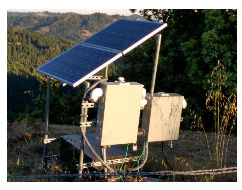
The posts are lengths of chain link fence top rail and are anchored in concrete and bolted to the sides of the battery box.
