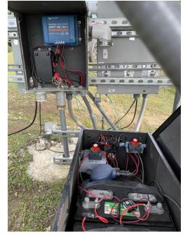
the radio. Previously, I would see the battery voltage drop below 12 volts after just a few minutes of transmission. A mobile radio's output power drops dramatically when the input voltage falls below 13.6v. With the booster, that is no longer a problem.
